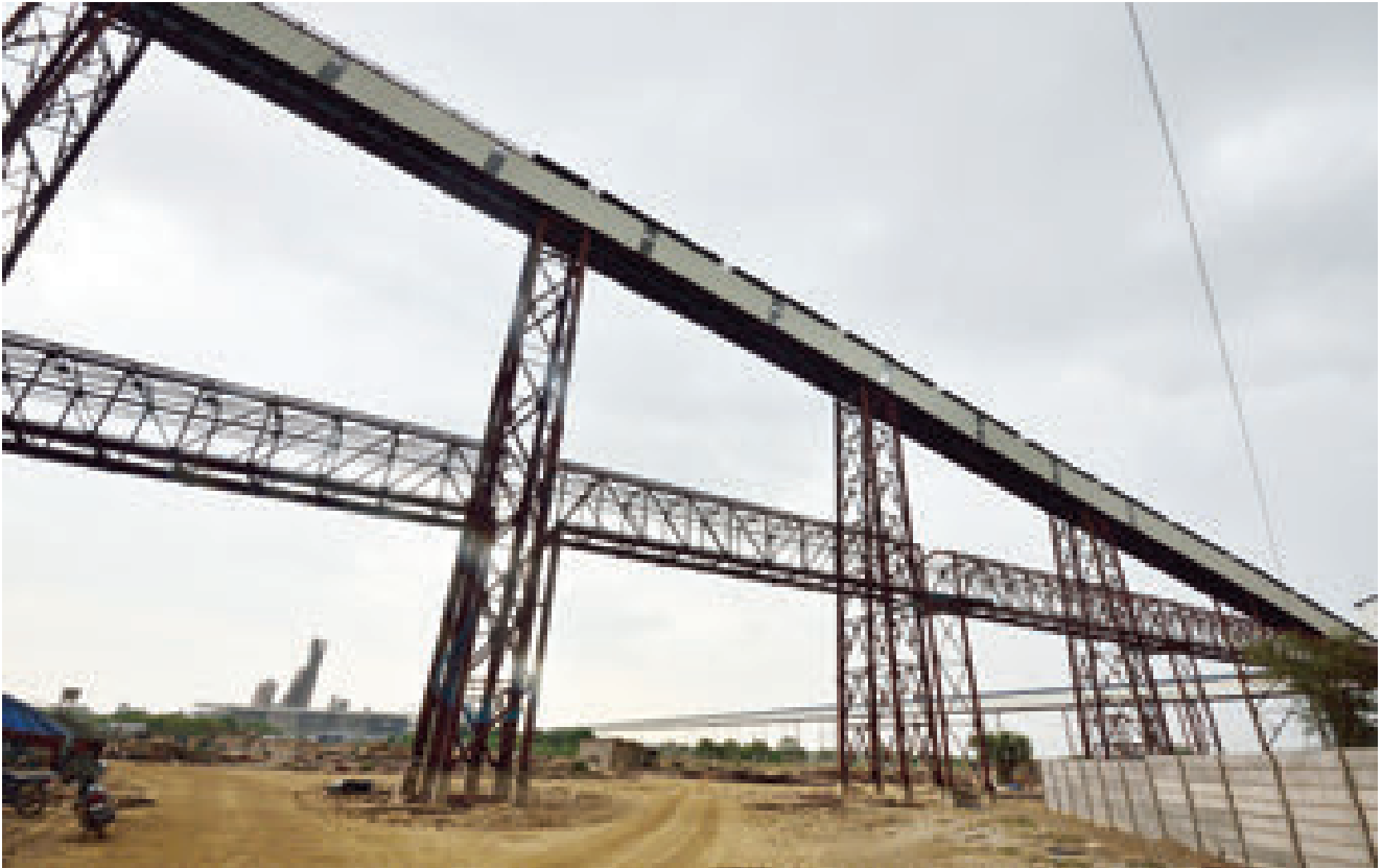
▲ Clinker transport to the cement mill by conveyor belt for seamless operations
