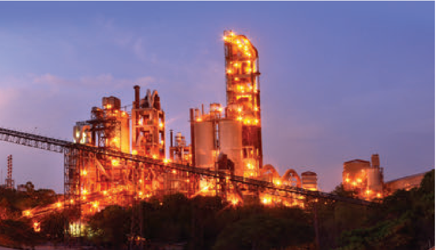
▲ View of the plant lit up at night
